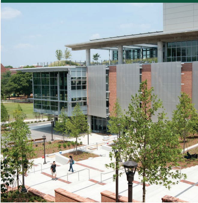
The LEED Platinum-certified G. Wayne Clough Undergraduate Learning Commons at the Georgia Institute of Technology. Photo: Georgia Institute of Technology
