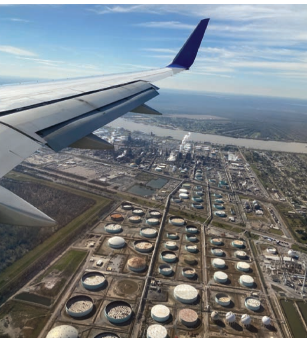
Industrial Infrastructure in New Orleans. Photo by Sarah Kallgren, NWF
