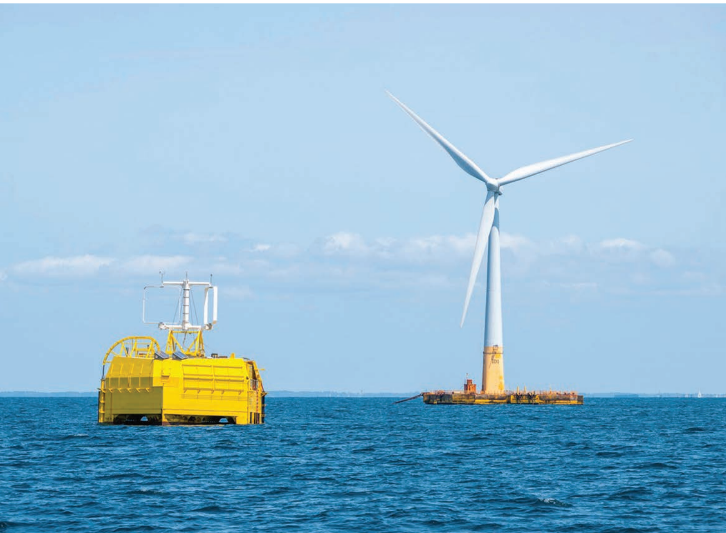
Sealhyfe offshore hydrogen production pilot (Lhyfe), on WAVEGEM platform (GEPS Techno) and floating turbine (BW Ideol). On the SEM-REV offshore testing site (Centrale Nantes / OPEN-C).
